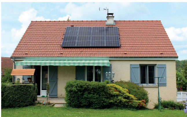
Torcenay 52600 - Panneaux photovoltaïques Viessmann
